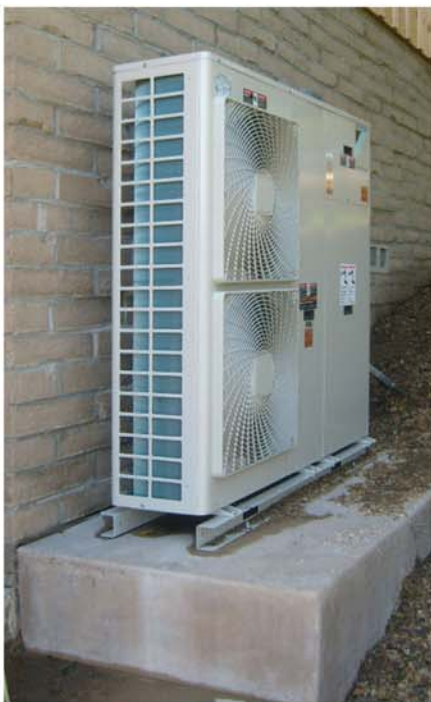
The very quiet Daikin Altherma air to water heat pump.
